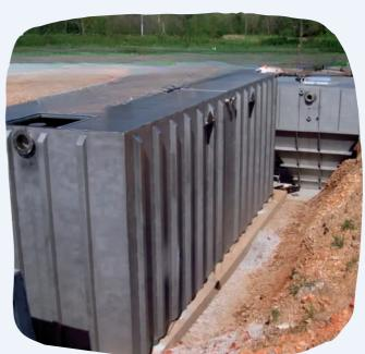
Contaminated water originating from domestic and industrial use is called wastewater. As wastewater content in domestic use is in a harmonious balance of carbon, nitrogen and phosphorus, we can make treated wastewater usable for garden and recreational field irrigation by applying physical, biological wastewater treatment systems and then filtration and disinfection system.
